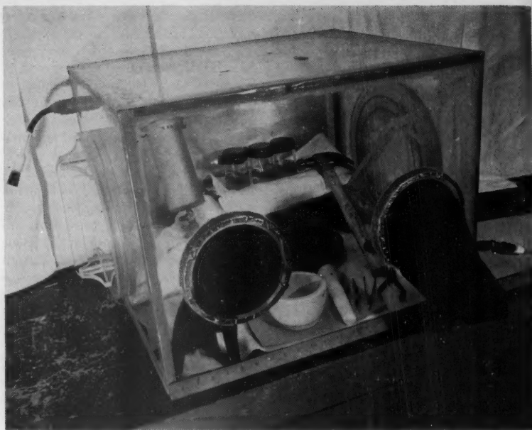
Fig. 1. Exposure chamber inside which electronic components are sterilized externally and then broken open so that they can be tested for internal bacterial contamination. A sterile hammer, anvil, pliers, and mortar and pestle may be seen, as well as the taped broth blanks into which the pieces from the components are placed. The empty ethylene oxide container is at the rear of the chamber, at left. The components to be tested are hidden behind the rubber gloves.
